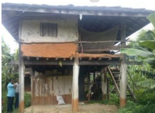
Figure 5: Typical timber framed house
