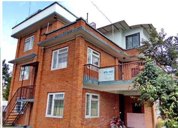
Figure 4: Typical brick in cement mortar house
