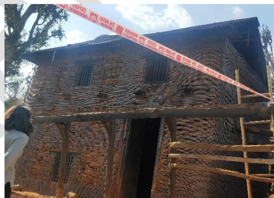
Figure 17: Retrofit of a house in splint and bandage approach
