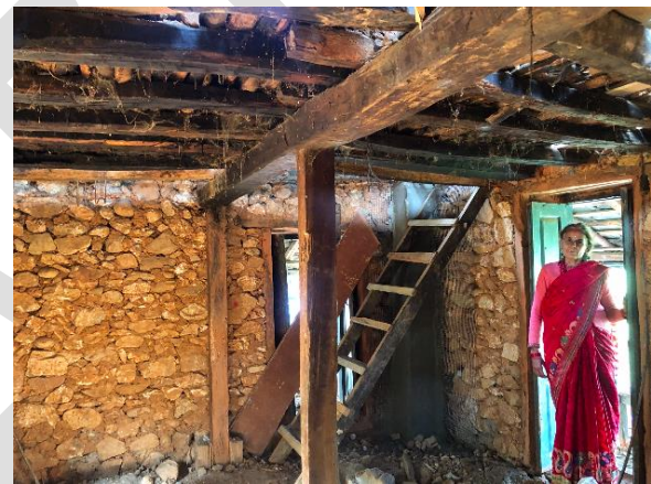
Figure 2: Ground floor room of SMM building
