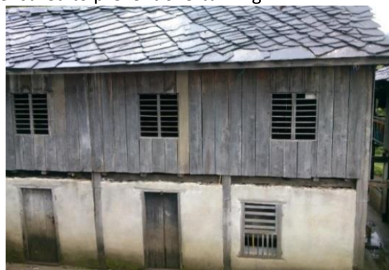
Figure 6: Typical timber frame building with masonry infill in ground floor
