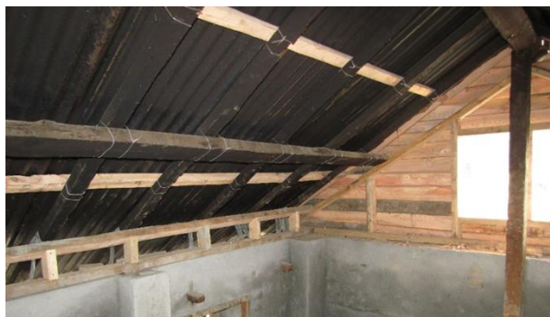
Figure 15: Improvement of existing timber connection
