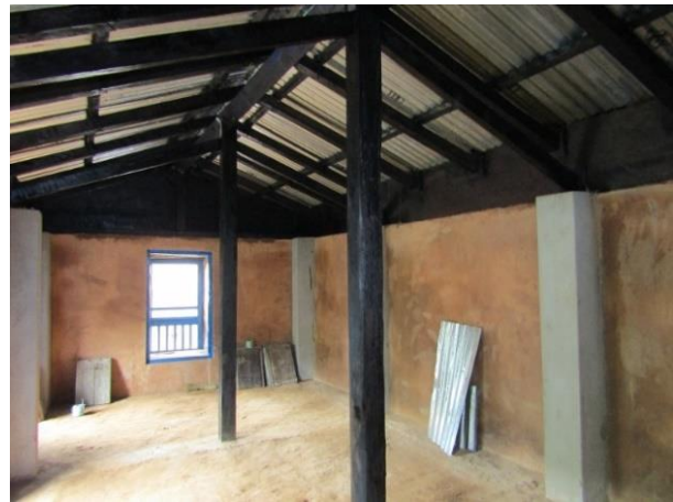
Figure 9: House retrofitted using the strong back approach
