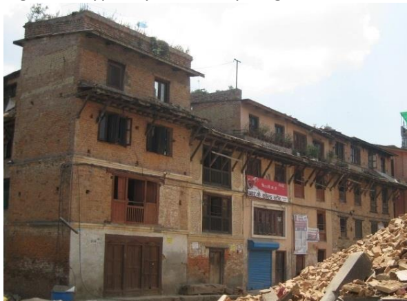
Figure 3: Typical brick in mud mortar house
